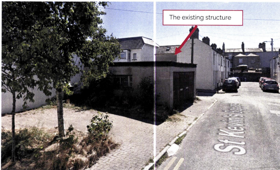
Fig. 3: The location and appearance of the existing structure within St. Kevin's Square – Google Streetview 2014
